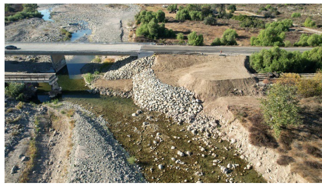
After: Emergency Repairs Complete – 10/24/2024
