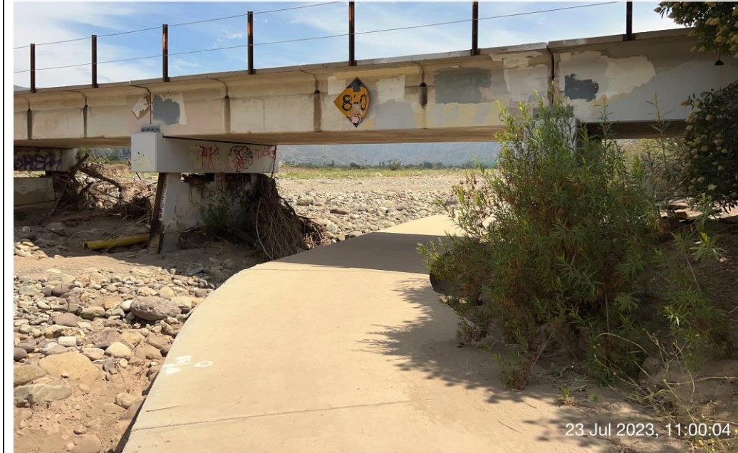
Photo 4. South abutment looking east
