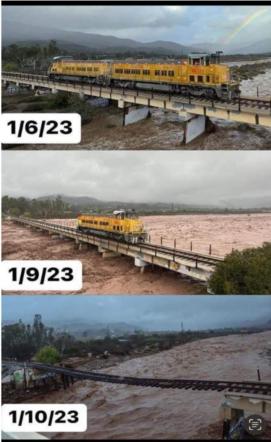
Figure 3. Photographs of VCTC Sespe Creek Bridge, January 2023.
