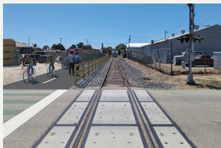
Exhibit 6. Railroad corridor with trail in confined ROW through Saticoy
