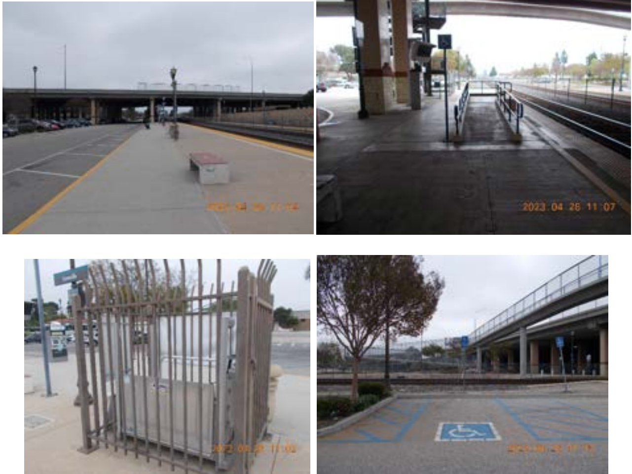
Figure 5. Site Photos of existing Camarillo Station
