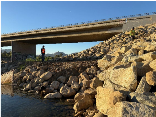
Illustrative photos of Emergency Repairs to Stabilize West Embankment of Sespe Creek Overflow railroad right-of-way.
