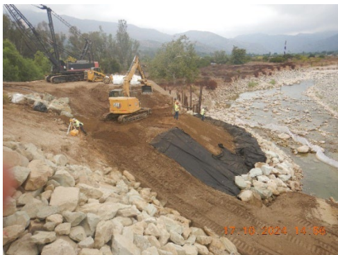
Illustrative photos of Emergency Repairs to Stabilize West Embankment of Sespe Creek Overflow railroad right-of-way.
