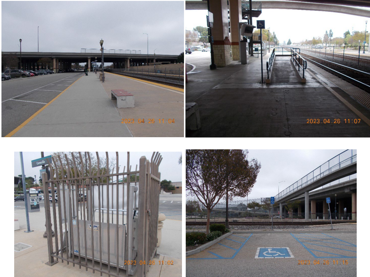
Figure 5. Site Photos of existing Camarillo Station
