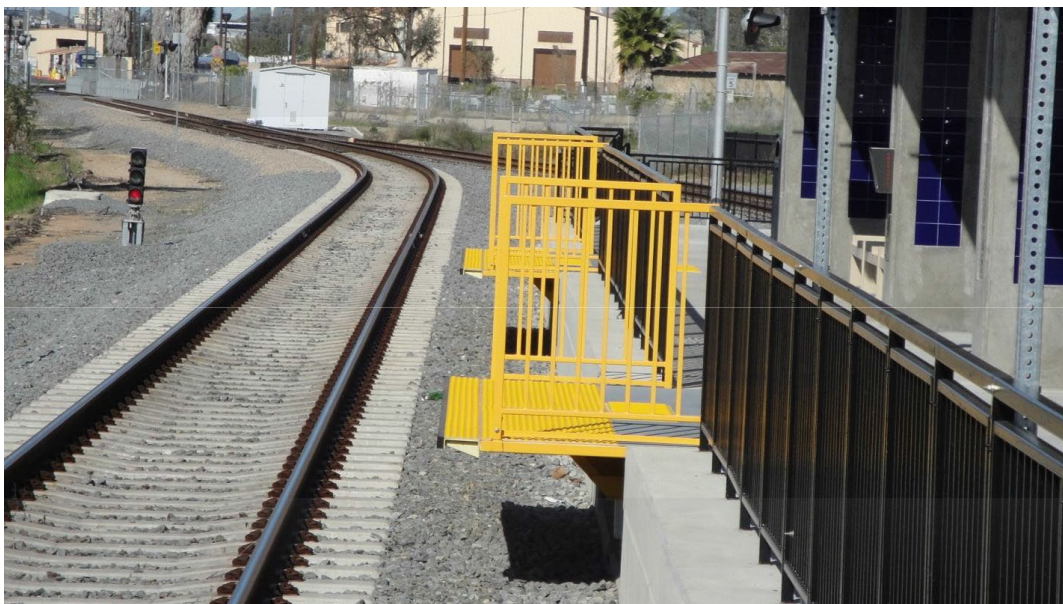
Figure 26. Station-based Retractable (Flip-up) Platform Edges
