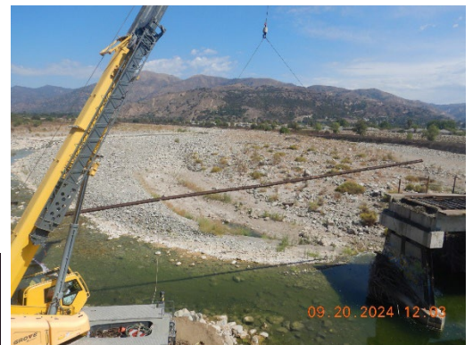
Removal of suspended railroad ties and rail by crane.
