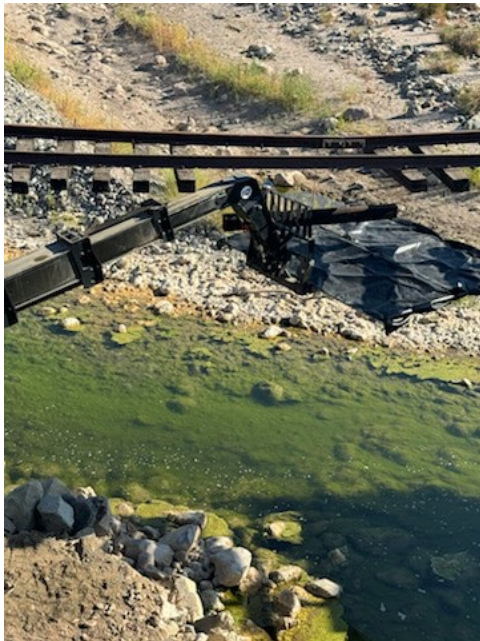
Removal of suspended railroad ties and rail by crane.
