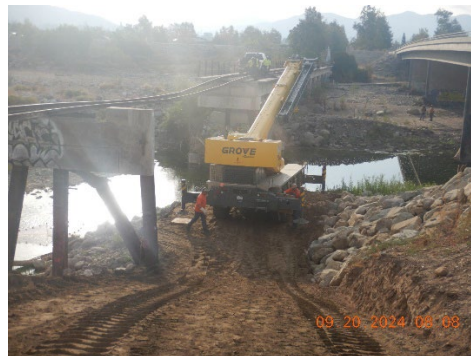
Removal of suspended railroad ties and rail by crane.
