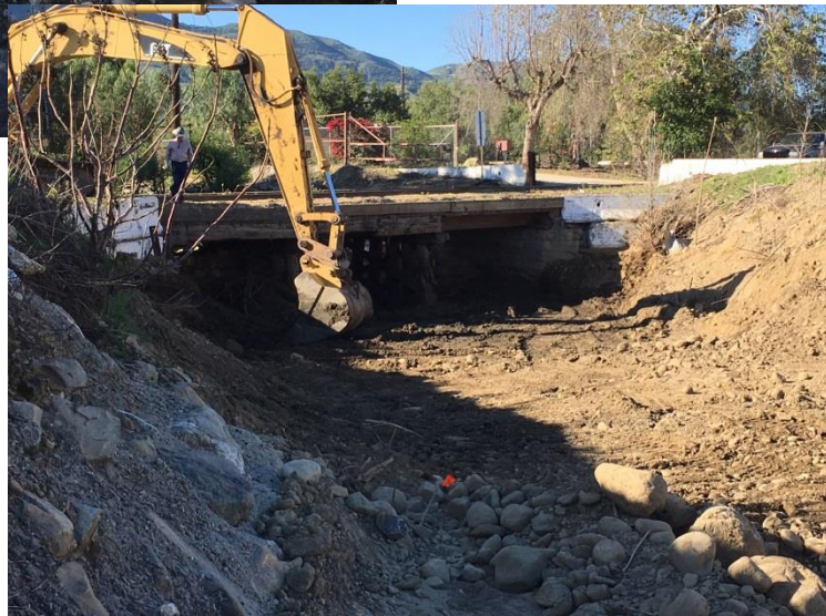
Haun Creek Bridge March 29, 2017
