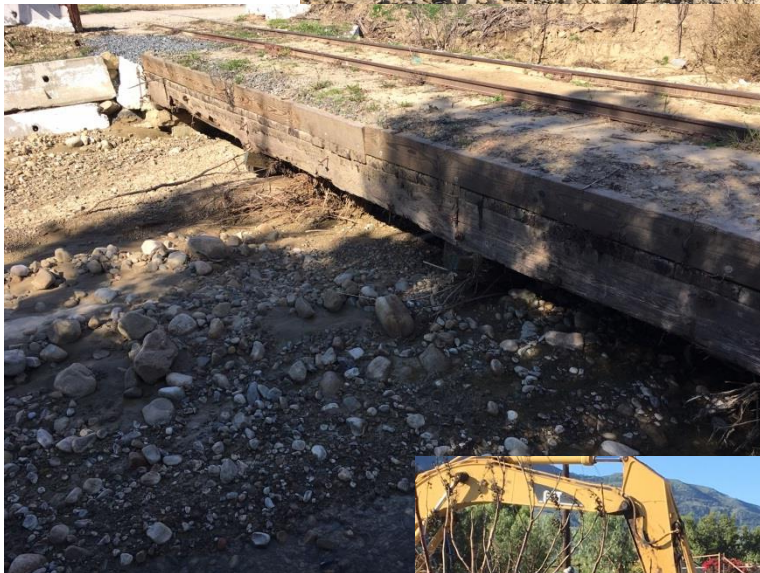
Haun Creek Bridge March 2, 2017
