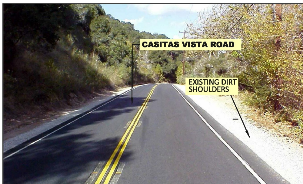
CASITAS VISTA ROAD - EXISTING CONDITION
